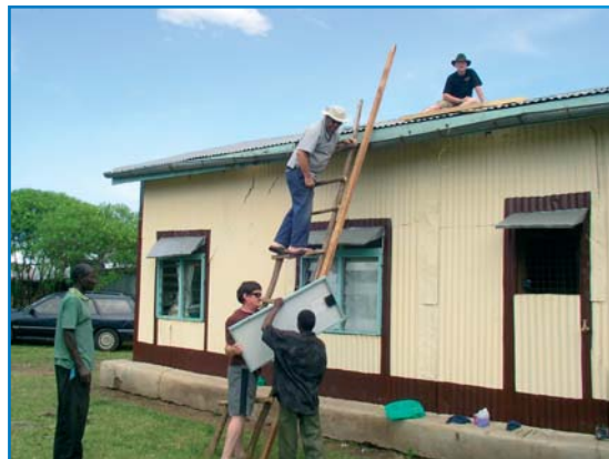
Installing the solar panels using a hand made ladder
